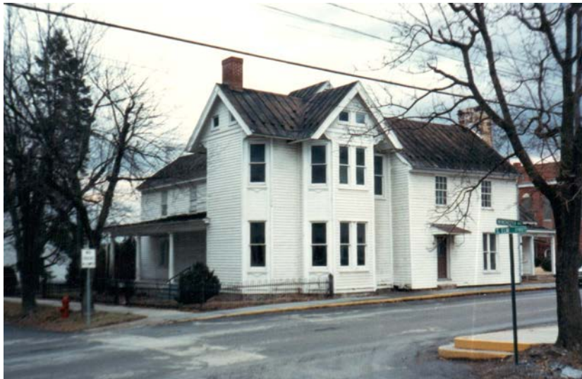
Higgins House is seen on far right of larger addition
