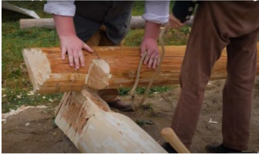
Timbers hand-notched for log cabin construction
