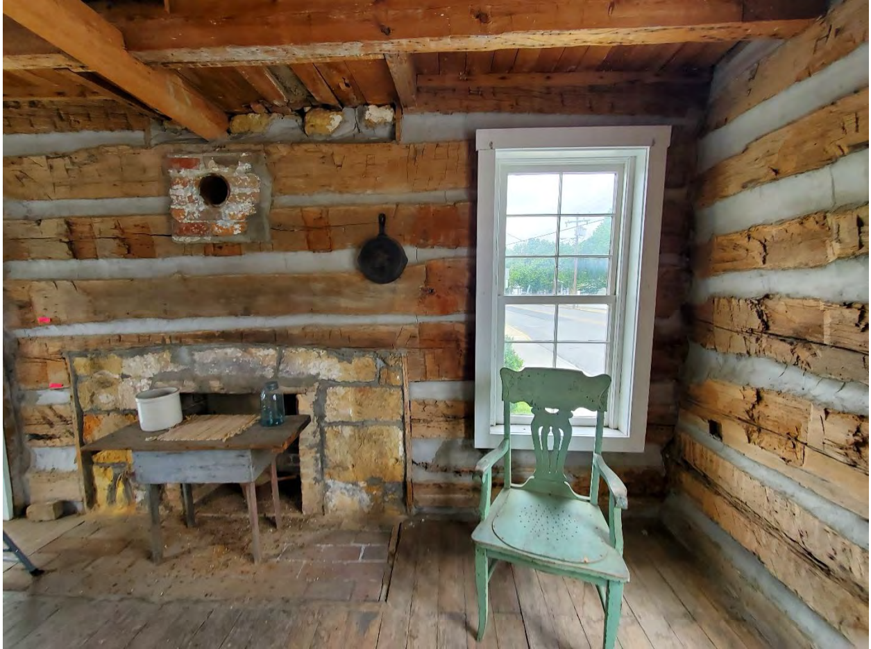
Figure 3. Logs are fully exposed on the interior of the Higgins House. View of first floor east wall (hearth) and south wall (to right).
